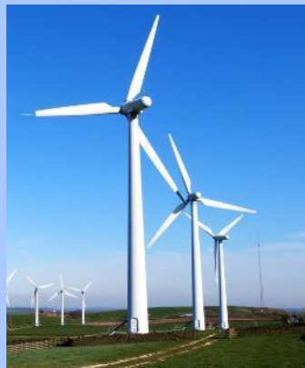
Wind power generator
