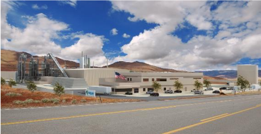
Biorefinery (under construction)
