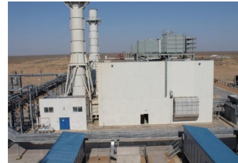
APG-fired power plant based on 3 x H-25 in Kazakhstan
